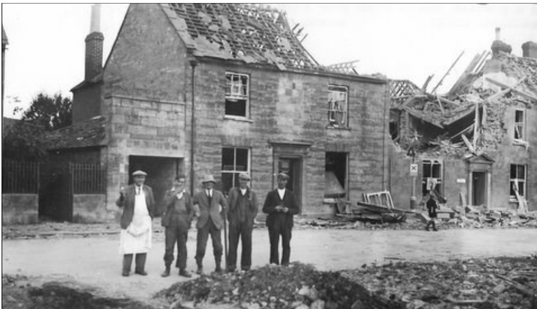
HERE IS THE NORTH SIDE OF NEWLAND FOLLOWING THE BOMBING RAID AND INSET ON THE RIGHT—TODAY.
