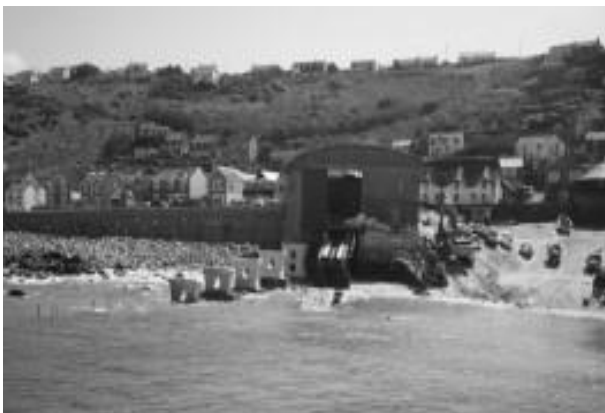
The Sennen slipway under construction
